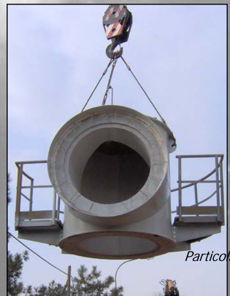
Finale combustore rivestito in materiale refrattario; Final part of combustion plant lined with refractory materials.
